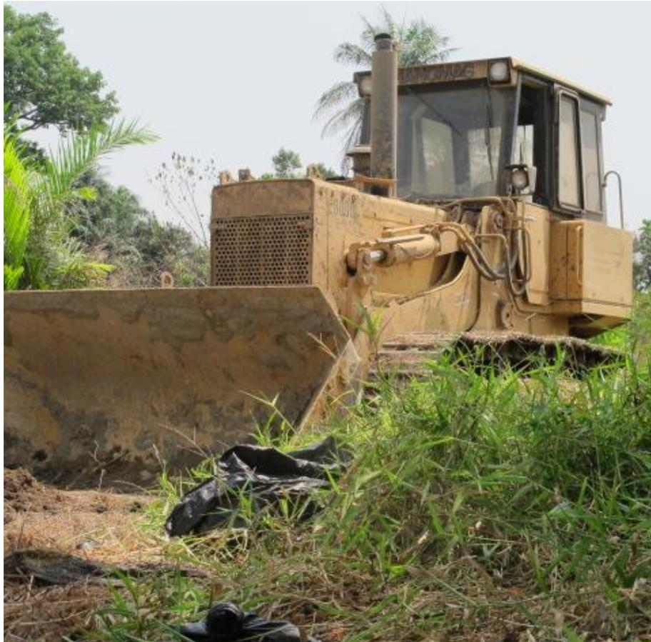
After drilling, section registration and sampling, the worked out cavity was back-filled with material in reverse way: Ballop → gravel → sand → clays → topsoil
